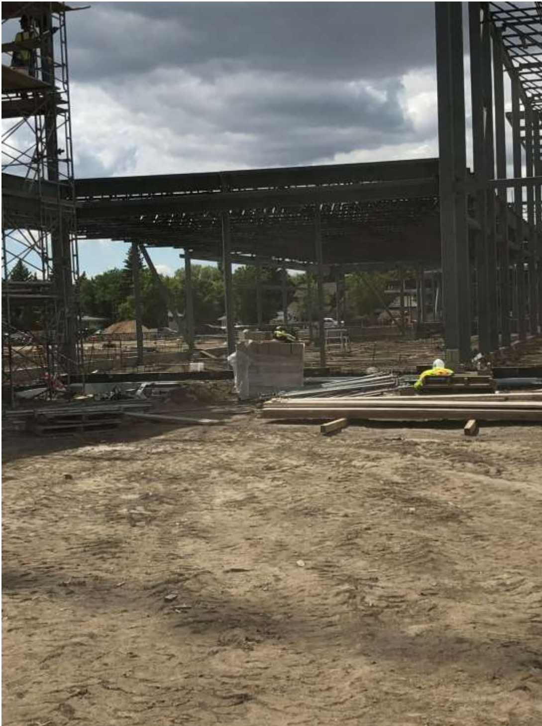
View from East to West from green space towards common area.
