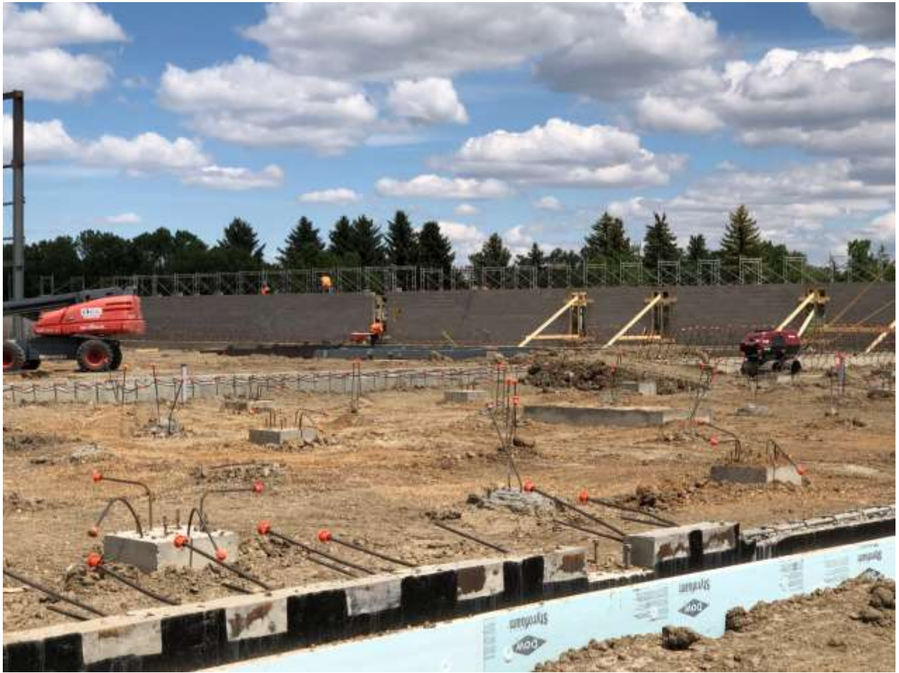
View from South towards East Change rooms / structural outer wall.
