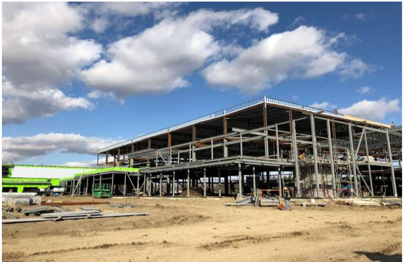
WRCC Front Entrance from Parking Lot
