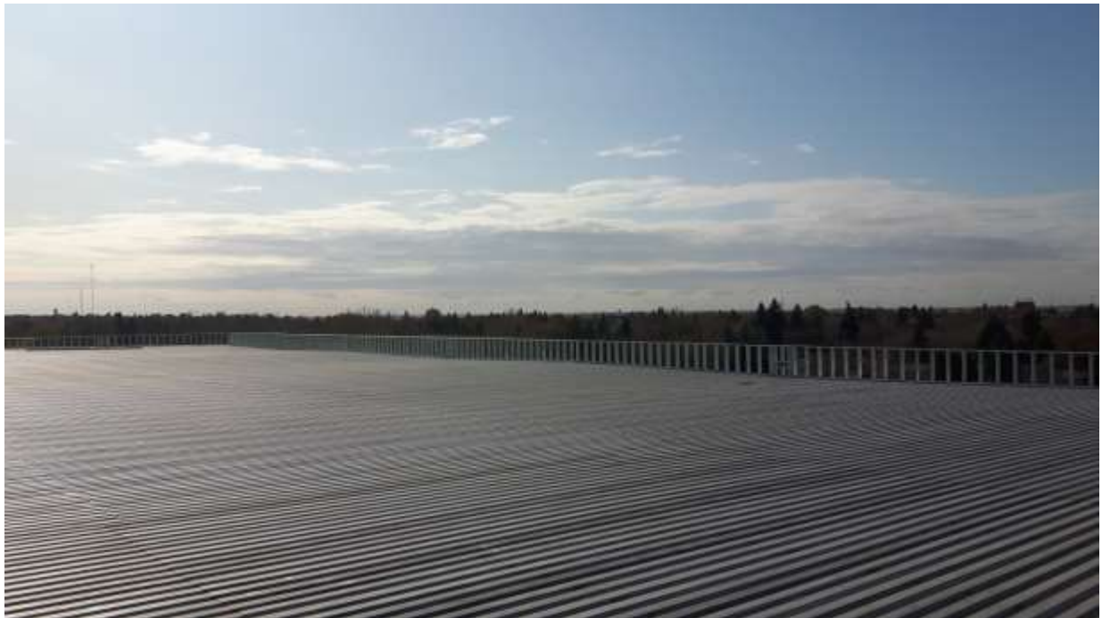
WRCC Roof Decking
