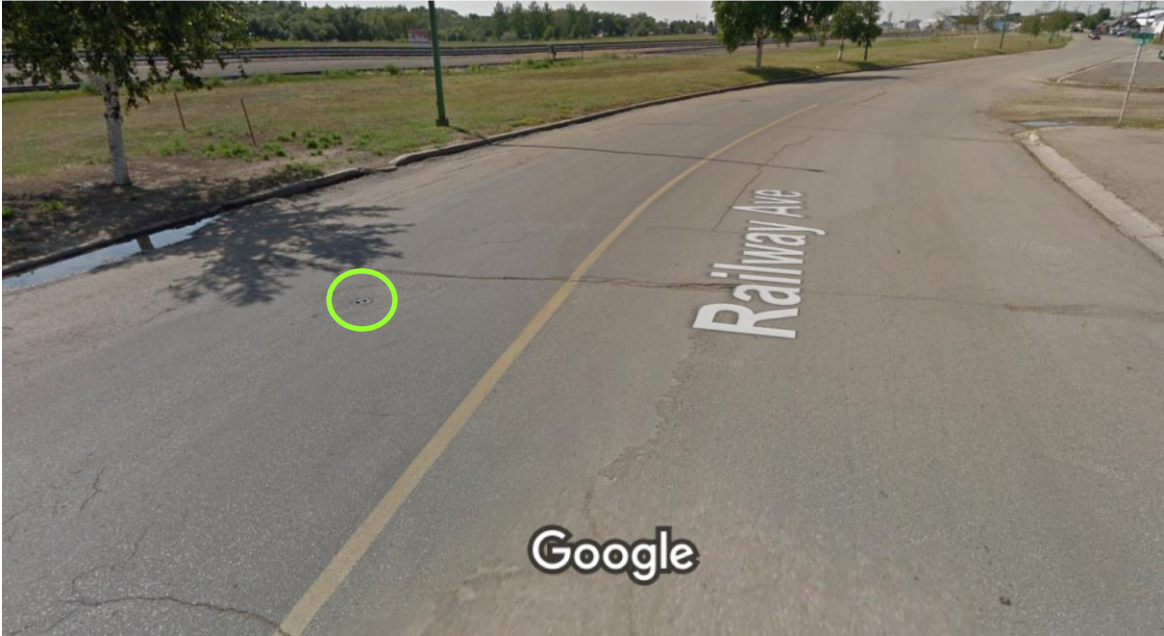
Figure 5: Railway Avenue and 10 th Street - Valve # 715
