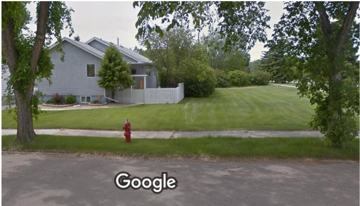
Figure 4: 11 th Street and 1 st Avenue NE - Hydrant # 38
