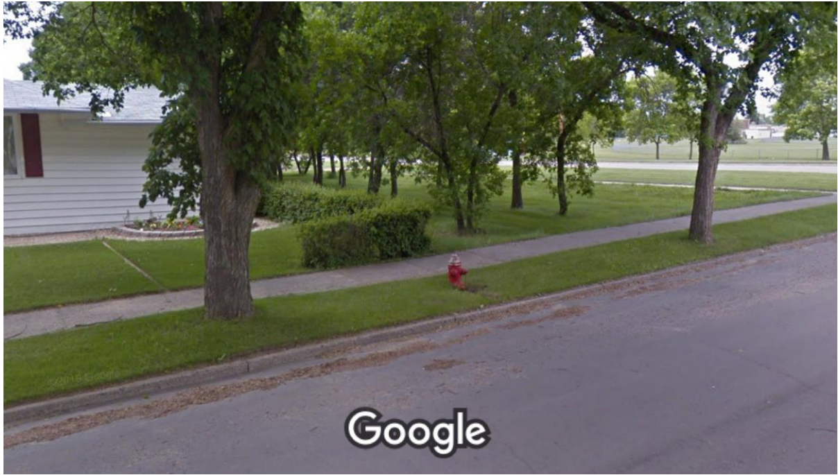
Figure 3: 10 th Street and 1 st Avenue NE - Hydrant # 37
